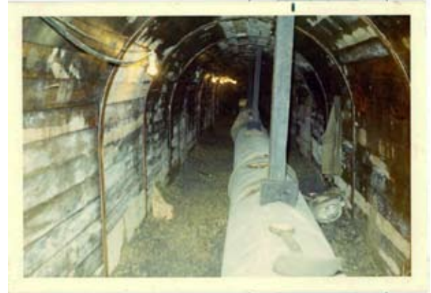
Inside the original sewer tunnel during construction, 1971.
